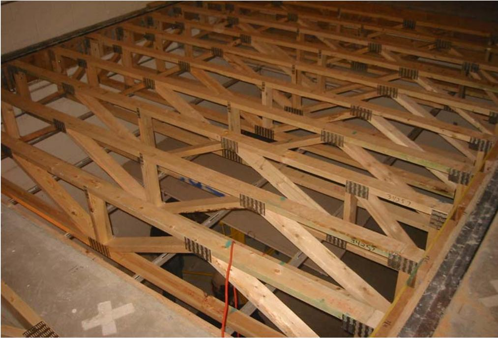
Figure 1: open-web trusses
