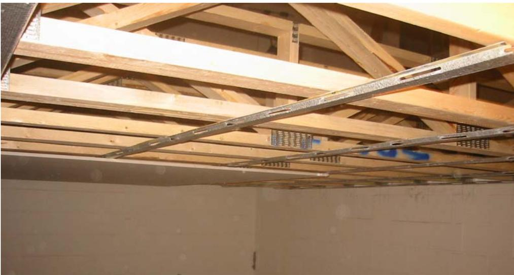
Figure 2: resilient channel and partial gypsum board ceiling
