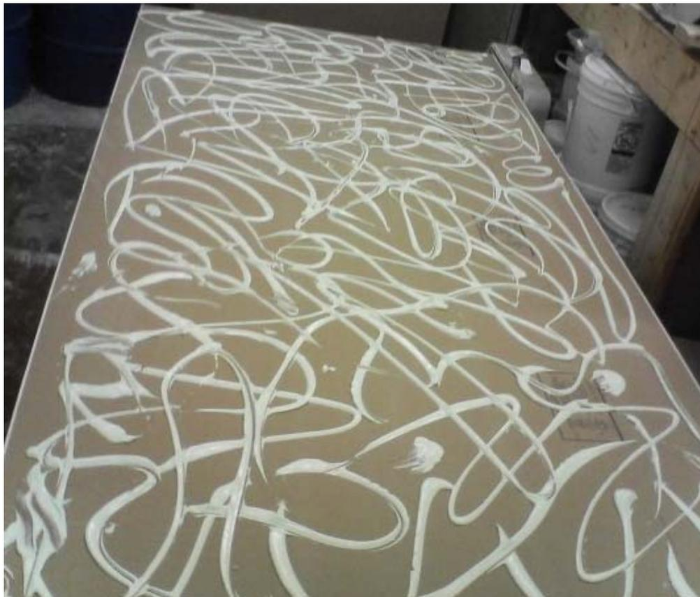
**Figure 1: Typical Green Glue Application (photo by client)**
